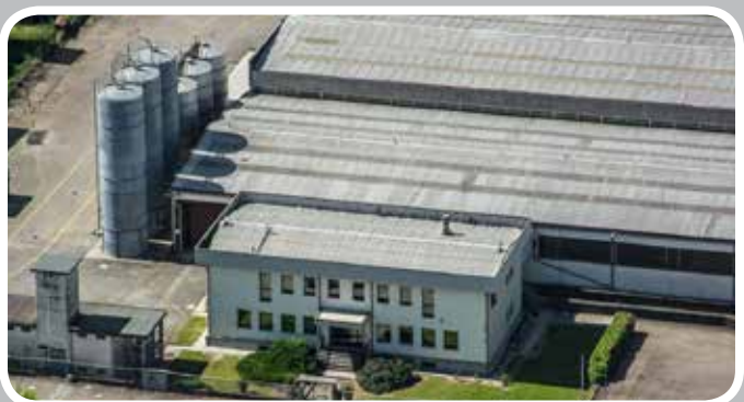
Production Centre - Imola (BO) - Italy
