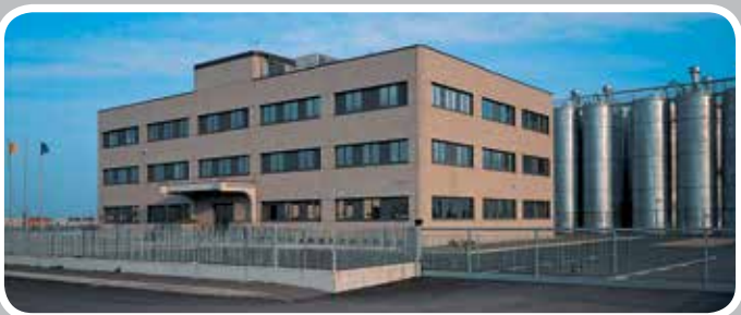
Production and Operations Centre - Castel Guelfo di Bologna (BO) - Italy
